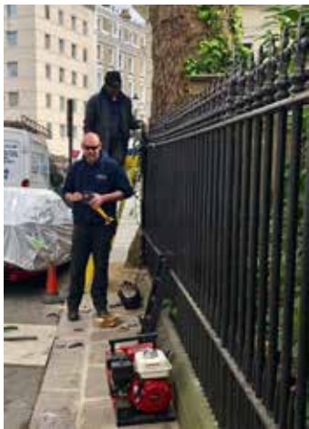
Railings specialists were hired to seal the opening.
